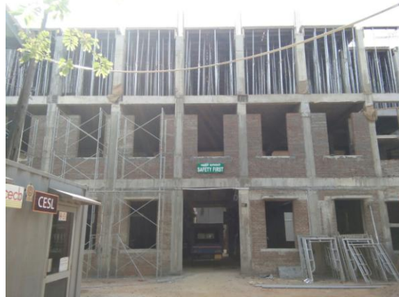
Anuradhapura Court Complex
